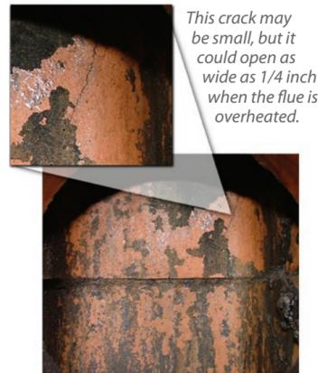
This crack may be small, but it could open as wide as 1/4 inch when the flue is overheated.
